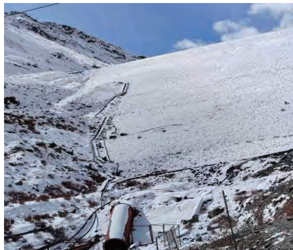
Figure 12.4: Downstream dam slope
