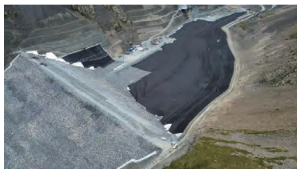
Figure 12.6: Ongoing construction – new TSF
