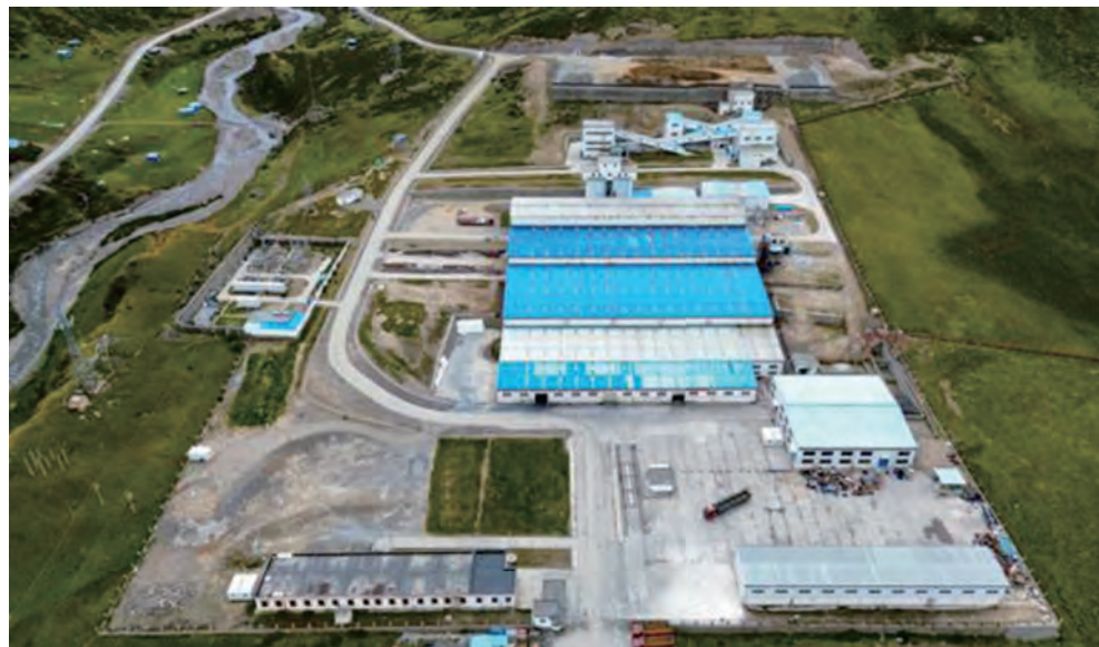
Figure 11.1: Drone photograph of the Mengya'a processing plant
