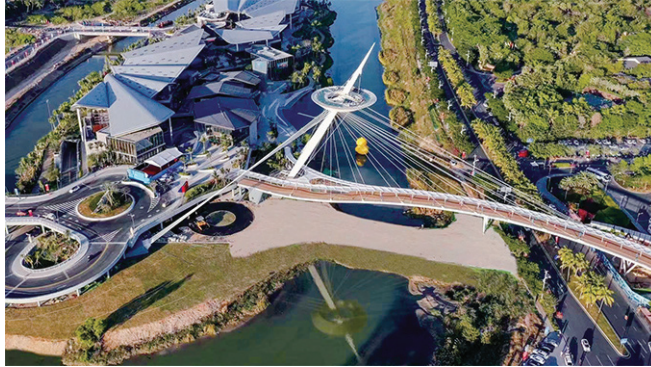
Landscape bridge connecting Phase II to Phase I
