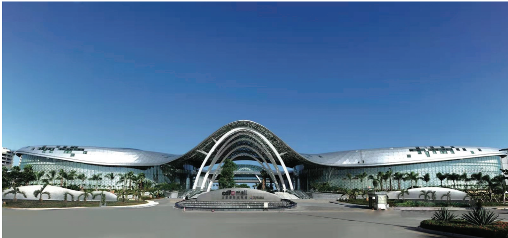
Exterior of Phase I of Sanya International Duty-Free Complex (Frontal View)
