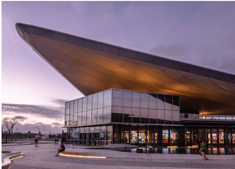
Exterior of Phase II of Sanya International Duty-Free Complex
