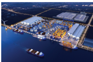
Hebei Tangshan Caofeidian Offshore Facility
