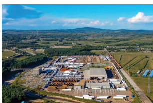
Liaoning Fuxin Onshore Facility
