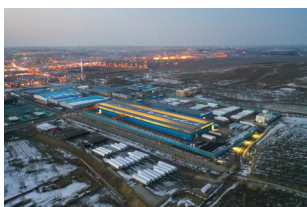
Hebei Zhangjiakou Onshore Facility
